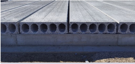
Figure 5 Precast hollow-core foundation slabs DRIVEN MICRPILES FULL SCALE LOAD TESTS
