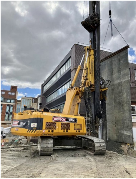
Figure 5 Close Proximity Piling
