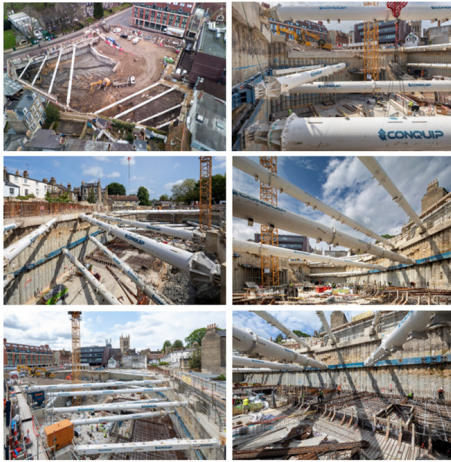
Figure 7 Basement Excavation & Propping
