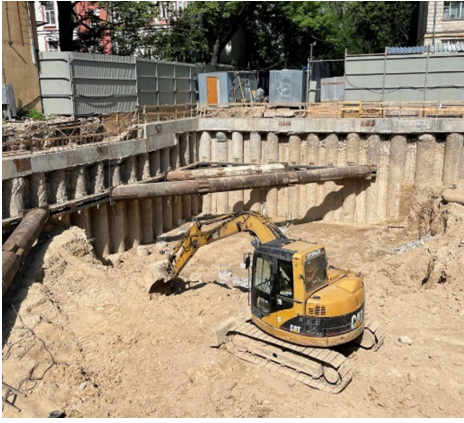
Figure 2 Construction site and retaining walls
